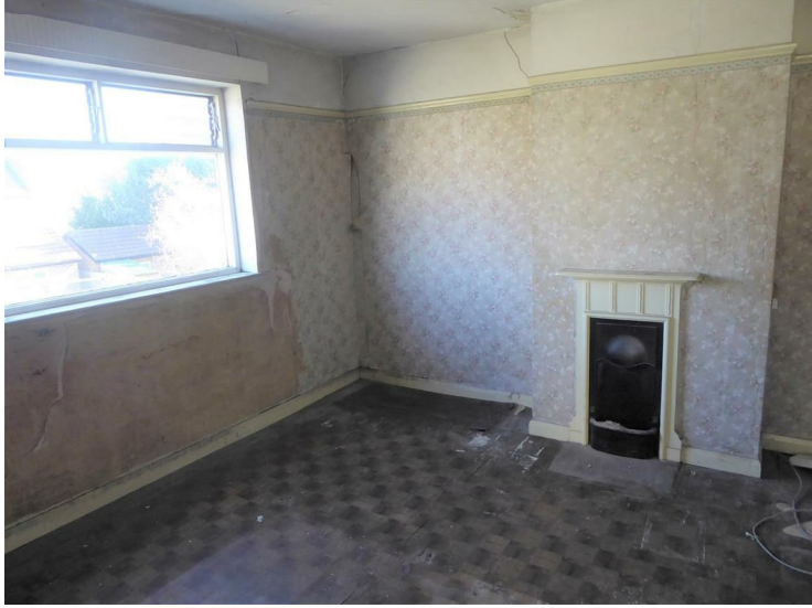
Rear aspect window, feature fireplace.
